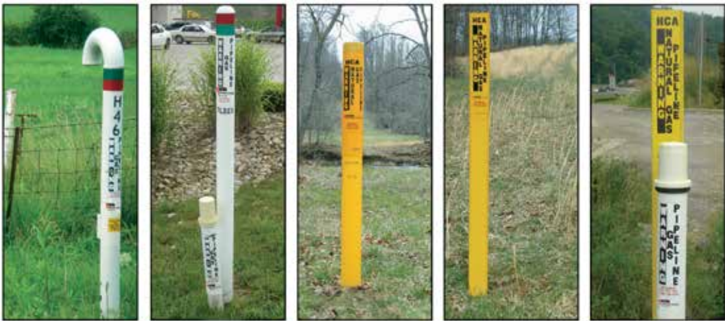
1. Vent Pipe 2. Linemarker and cathodic protection test station 3. High-consequence area entrance or exit marker (arrow on top) 4. HCA line-of-sight marker 5. HCA marker and cathodic protection test station
